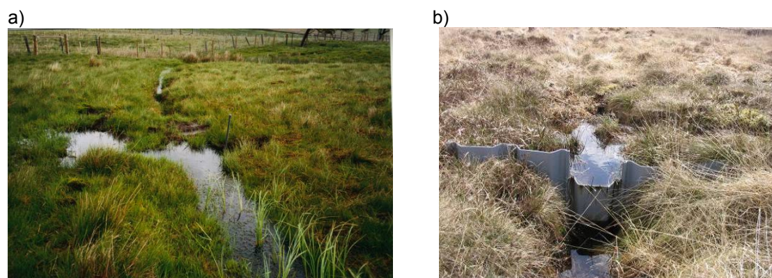
Figure 8. Dams in grips where (a) allows water to escape and rewet the general peat mass while (b) simply allows water to flow over the dam and back into the grip downslope. (Source: (b) courtesy of Dr Alona Armstrong)
