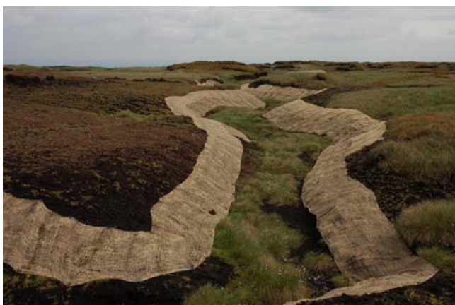
Figure 6. Geo-jute used to stabilise the peat in the Peak District
