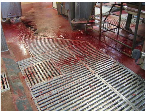
Figure 3A: Area of abattoir discharging into 6mm drainage trap
