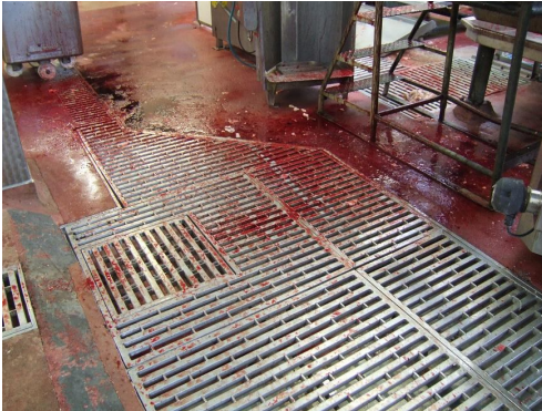
Figure 1A: Grids on abattoir floor to retain large fragments of carcass from drainage
