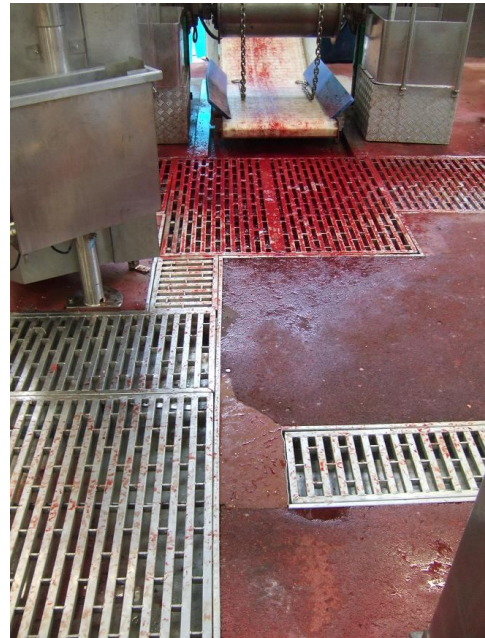
Figure 4A: Dividing line for wastewater in abattoir, to the right to blood tank and left to 3mm trap
