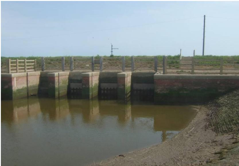
**Figure 3. New sluices have been installed to the west of Cley marshes to allow more rapid floodwater evacuation. Photo courtesy of Environment Agency**
