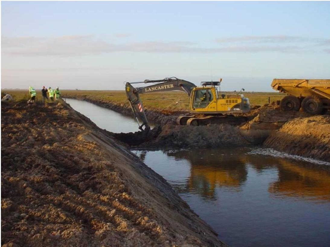
**Figure 5. Digger linking the final section of channel. Photo courtesy of Environment Agency**
