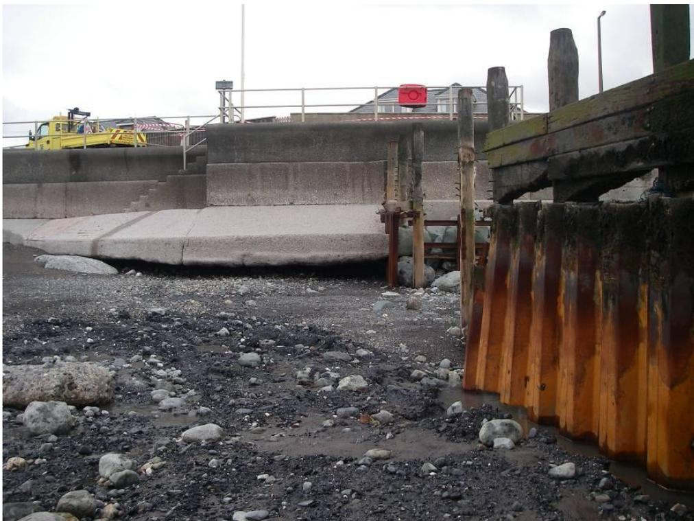
**Figure 3. Toe scour to sea defence at the promenade and dilapidation to groynes. Photograph courtesy of Gwynedd Council**
