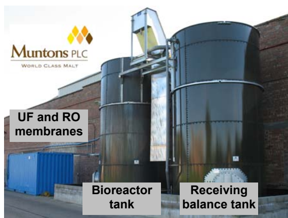
SWAN Commercial Pilot plant at Muntons plc, England. The two green tanks are 50m 3 each and the blue box housed the UF and RO membranes
