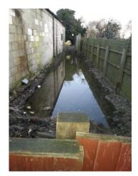
Trenches were excavated on three side of the farm building. Early problems with heavy rainfall caused problems with the trenches rapidly filling with water. The level of water in the trenches did dissipate over a period 10 days, suggesting that the system will work well as a SUDs reserve.
