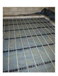
An underfloor heating system has been installed within the farm building with six diferent temperature zones. The building will eventually (depending on successful planning application) be used for demonstration and training purposes.
