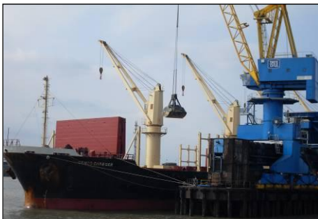
Jetty crane unloading at Thames Refinery
