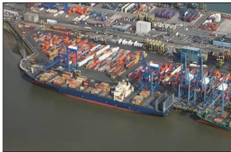
UK deep-sea container terminal (Tilbury)
